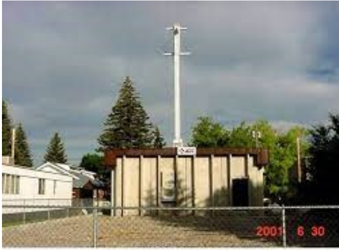
Mackay ATC Communications Building (Telephone and Internet) next to 413 Main June 30 2001
